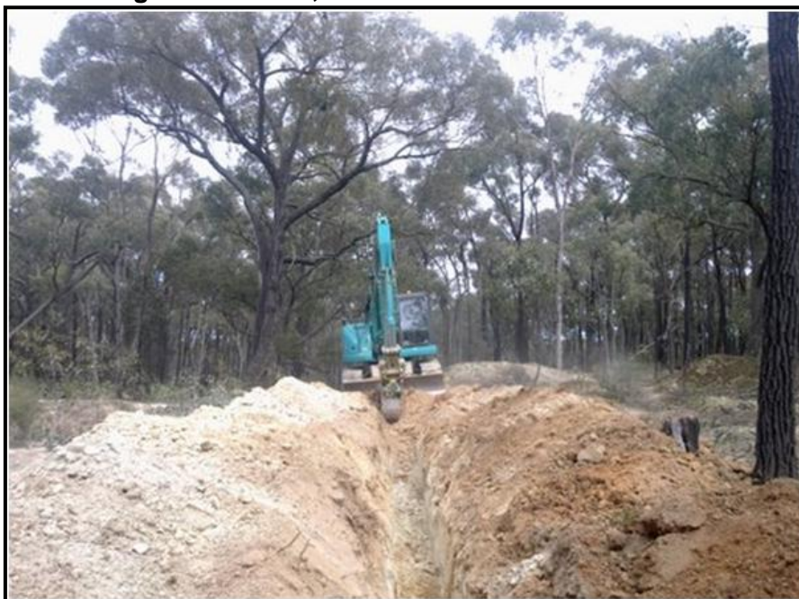
Costeaning at Redcastle, October 2011
