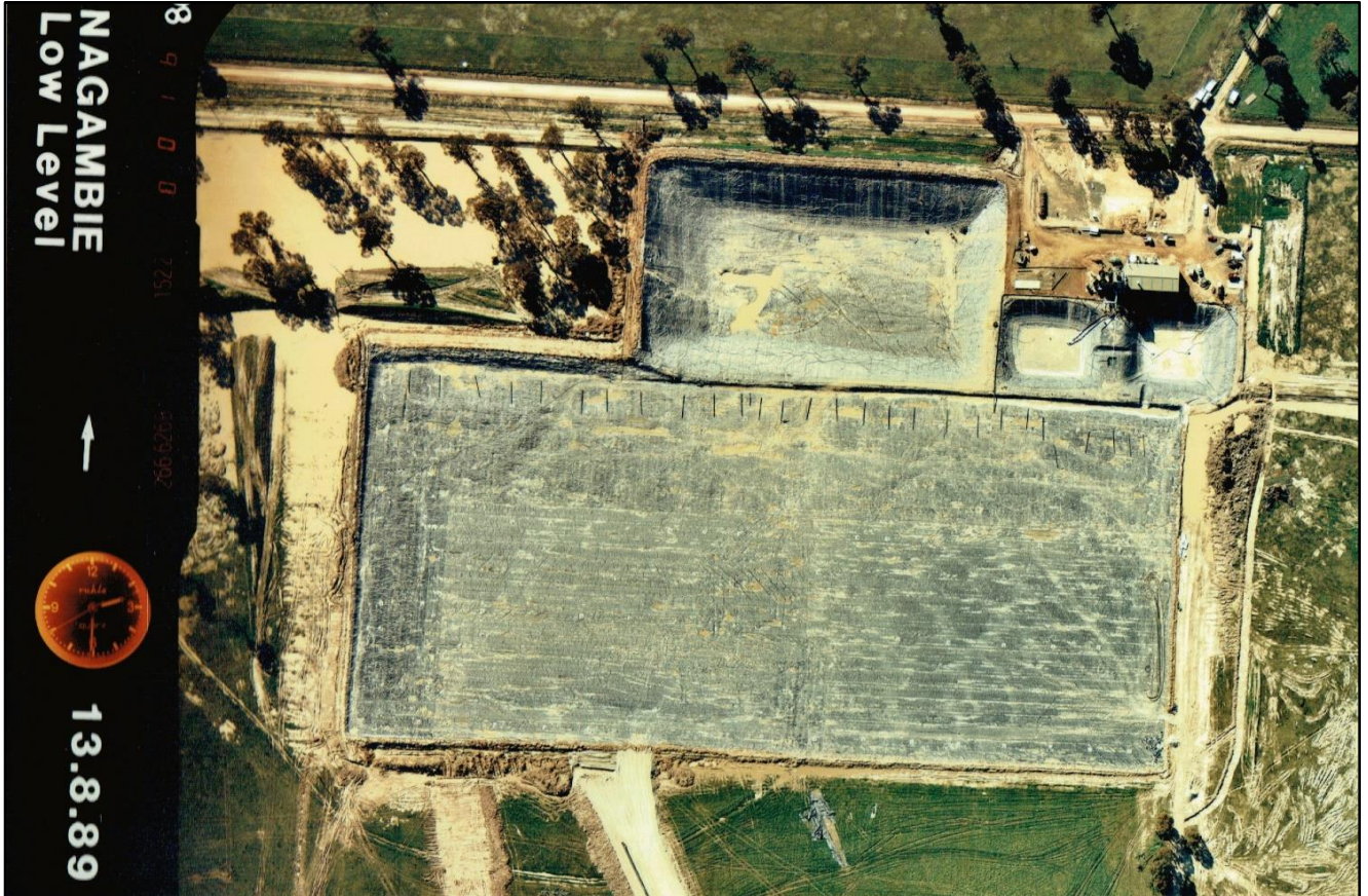
Photo 4 Aerial Photo of the HDPE Black Plastic Laid for the Heap Leach Pad and Ponds
