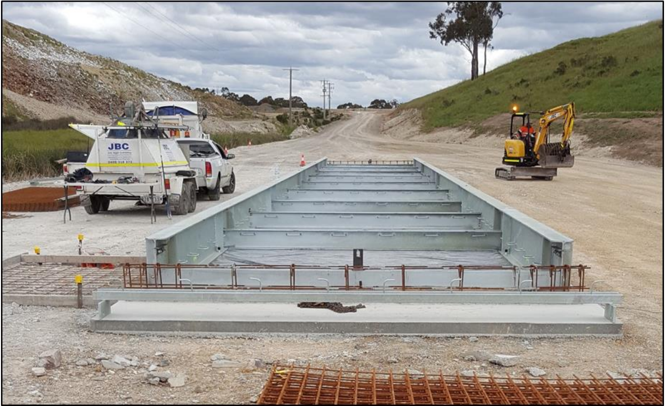
Photo 2 34m Weighbridge under Construction
