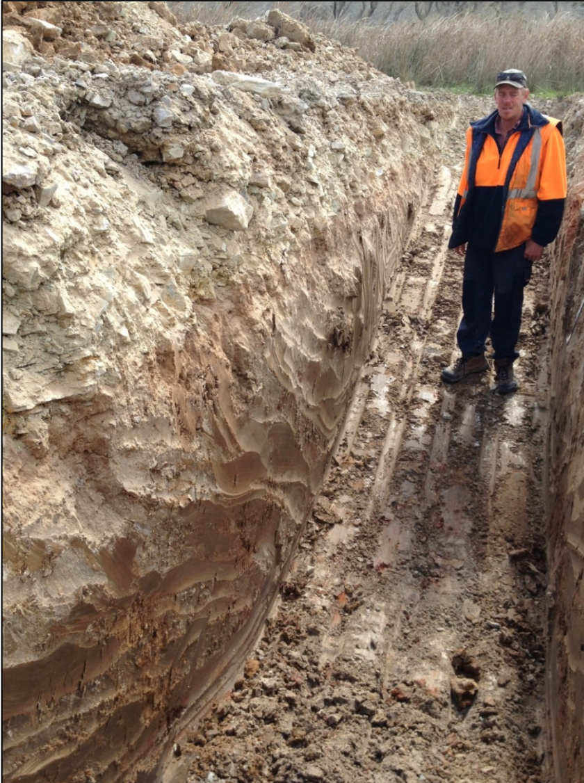
Impermeable surface clay that naturally lines the site
