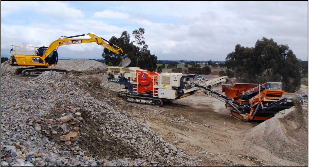
Photo 1 Global Excavator, Mobile Jaw Crusher and Mobile Screening Plant
