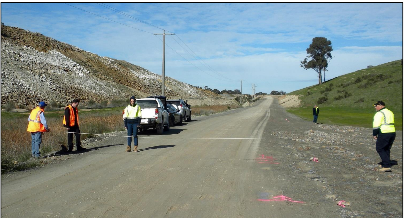
Measuring up the location for the Weighbridge
