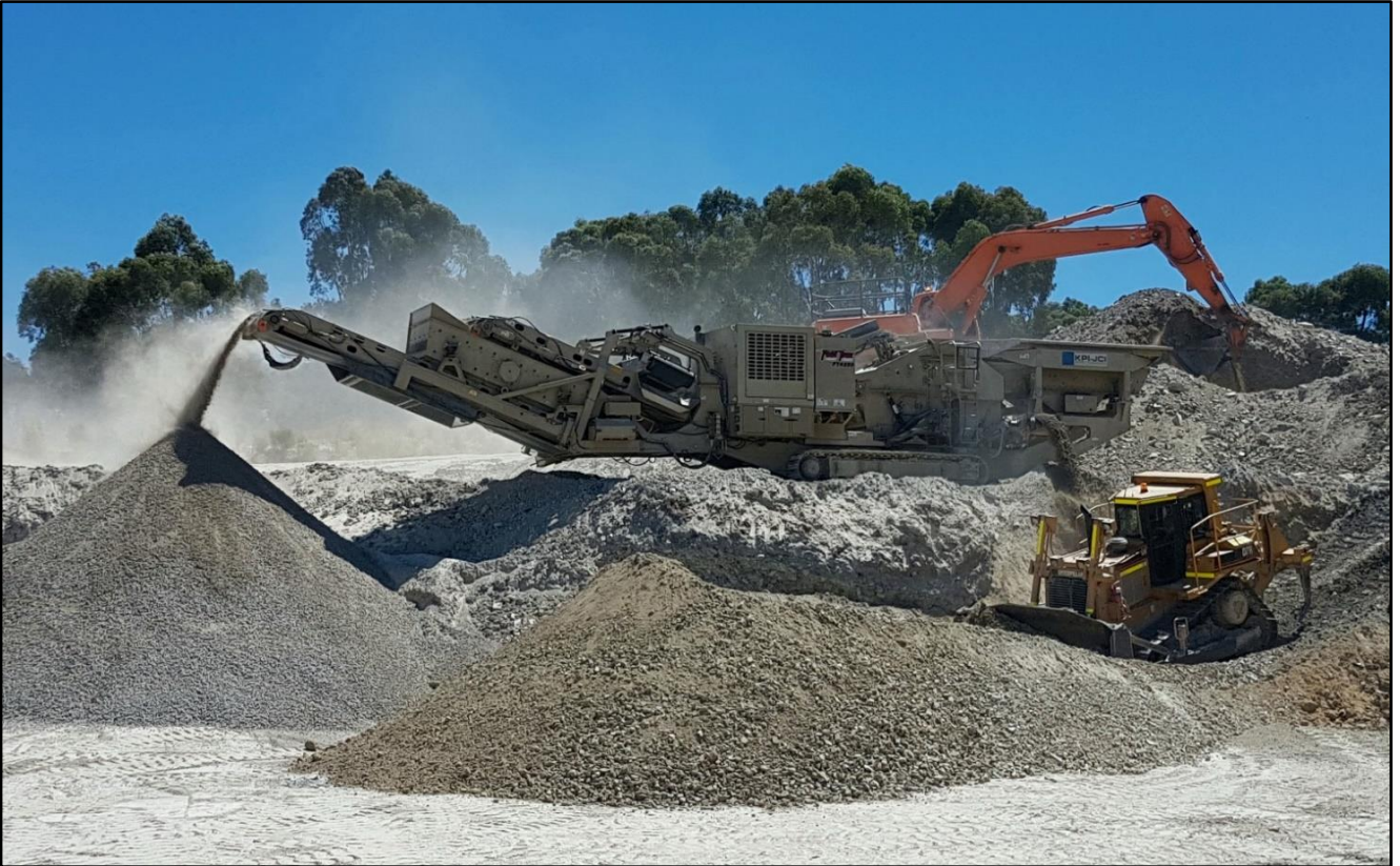
Photo 4 Crushing and Screening Unit in Operation at the East Overburden Dump
