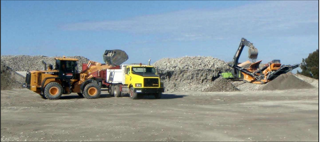
Photo 1 Global screening and loading crushed rock at the Eastern Overburden Dump
