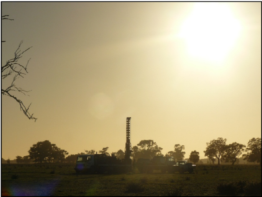
AirCore Drilling at Nagambie North, April 2011
